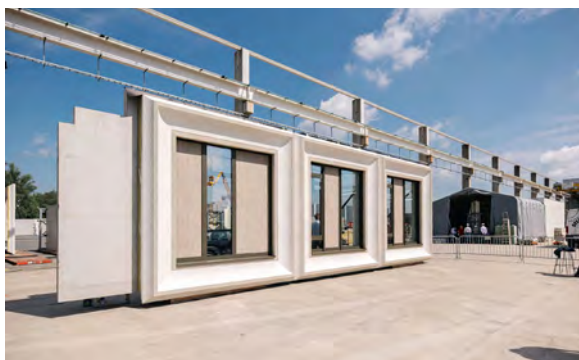
Façade frames of Hospital Jan Portaels in Brussels, Belgium, were produced using D-Carb by C-concrete.
