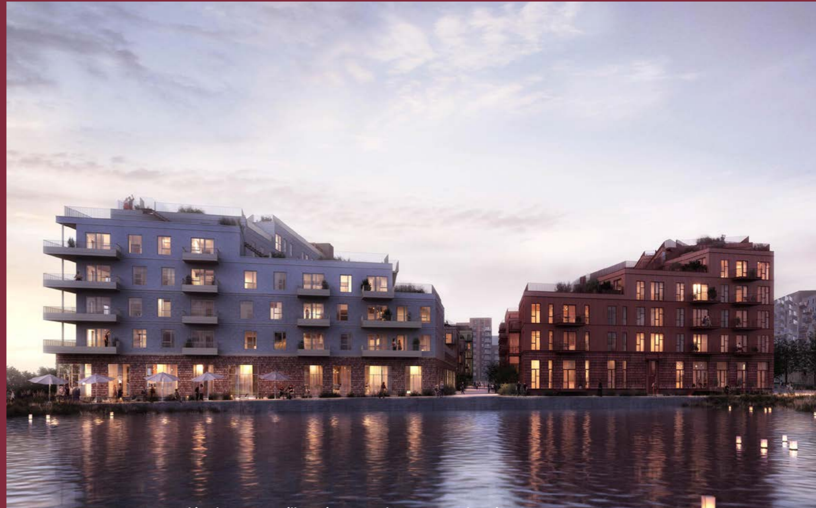
▲ FUTURECEM was used in the UN 17 Village in Copenhagen, Ready-Mix Concrete supplied by Unicon and managed by the construction company CG Jensen. The project designed by Sweco Architects and design layout by Lendager Group
