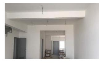
A sight to behold, White wall finishes on the apartments internal wall applying SCI Mortar White 853 for base coat and finishes with SCI Plaster White 855 in total 1,019sqm per unit at the 46storey Laurels Tower.
