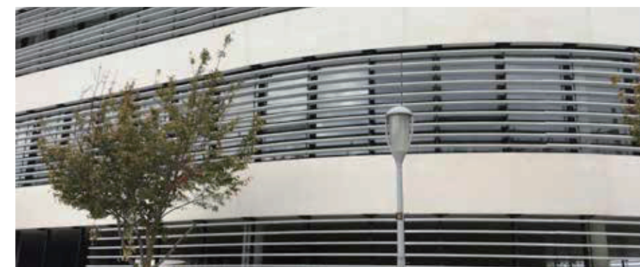
All elements are produced with the ultra high-performance concrete Aalborg Extreme® developed by Cementir's Innovation Team
