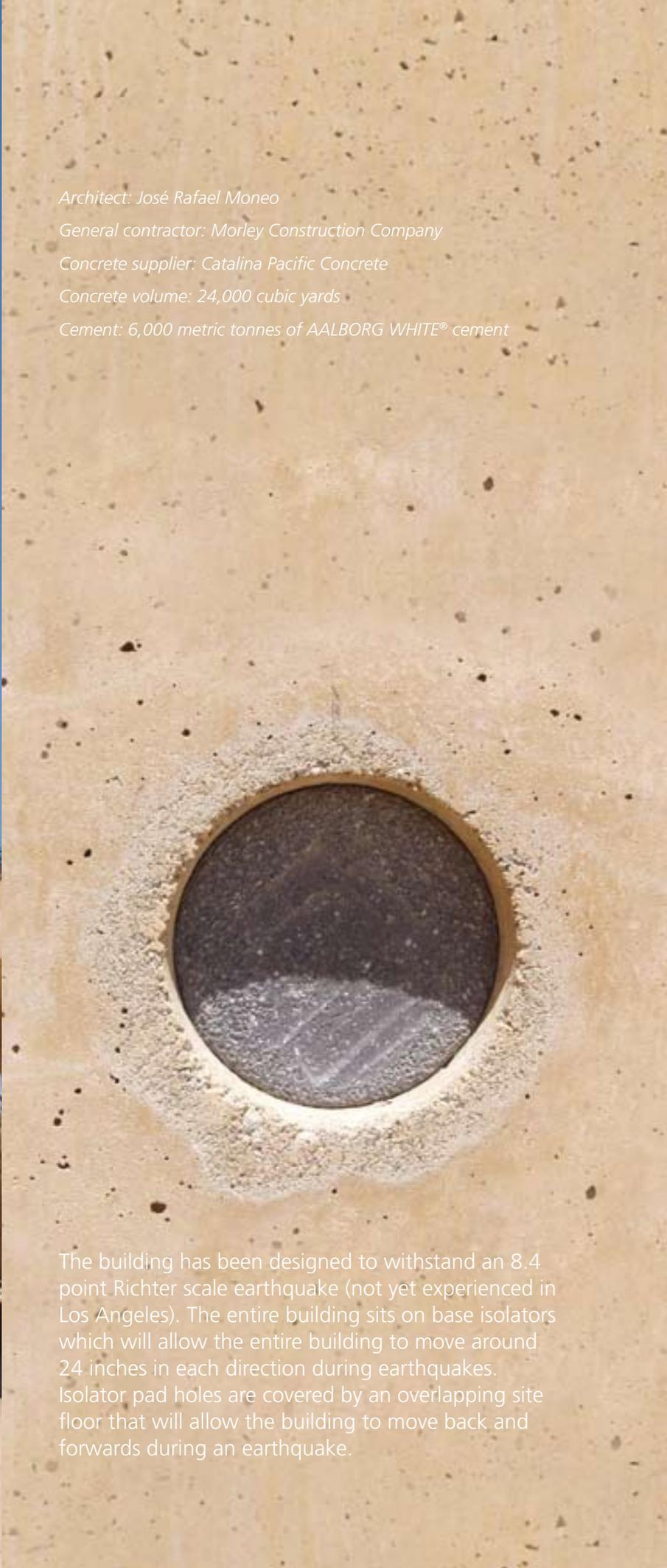
The building has been designed to withstand an 8.4 point Richter scale earthquake (not yet experienced in Los Angeles). The entire building sits on base isolators which will allow the entire building to move around 24 inches in each direction during earthquakes. Isolator pad holes are covered by an overlapping site floor that will allow the building to move back and forwards during an earthquake.
