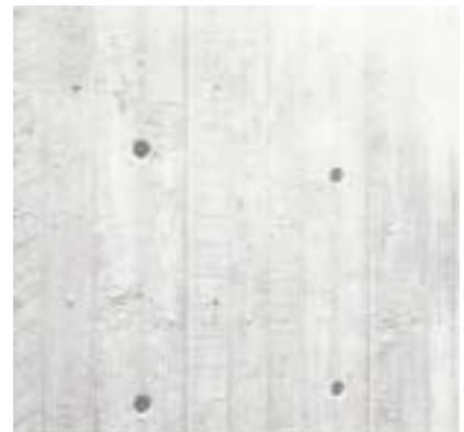
Concrete surface – from rough shuttering boards.
