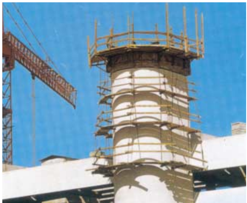
Sliding shuttering, Herlev Hospital.
