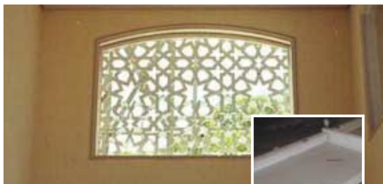
Surface from plastic formwork
