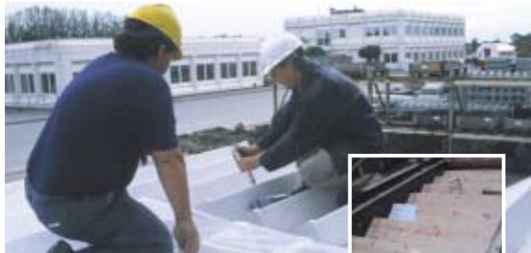
Surface from wooden formwork
