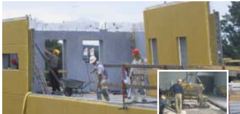
Surface from steel formwork
