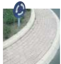
Clear marking with white concrete kerbstones.
