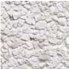
White exposed coarse marble aggregate after grinding, with retarder.
