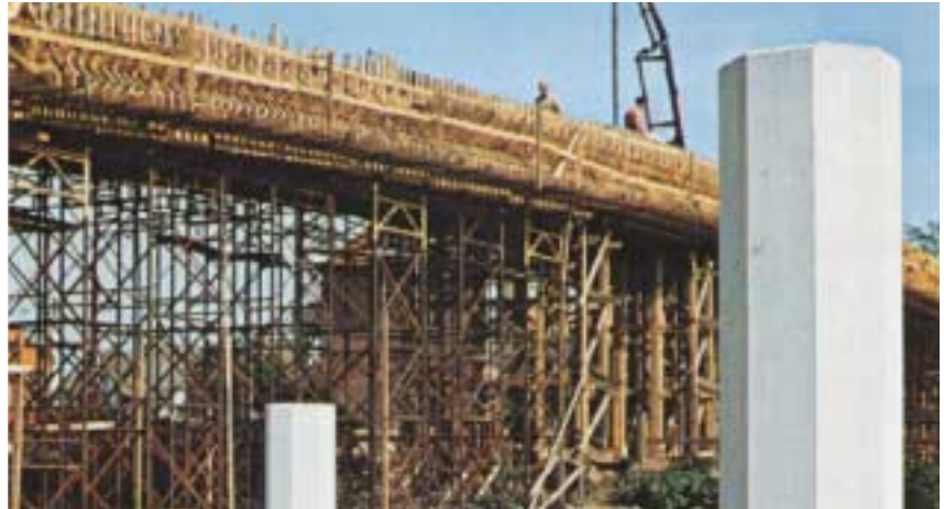
Shuttering for pedestrian and cycle bridge in white concrete.
