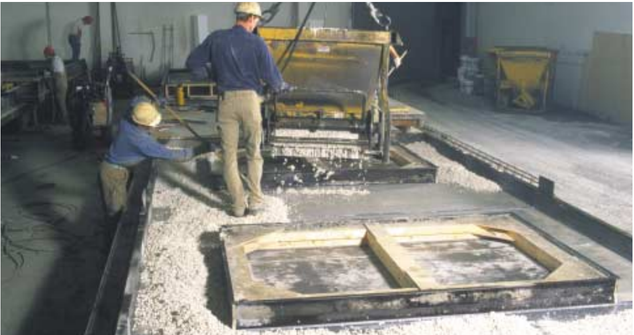
Vibrating table for concrete elements for facings.
