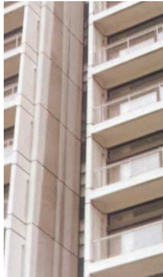
Dirt on a gable because of shadowing from a neighbouring gable.
