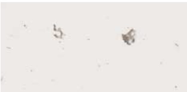
Example of pore formation from the incorrect choice or pre-treatment of formwork material.
