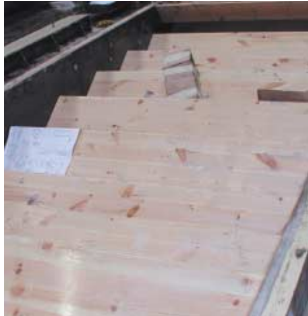
Wooden formwork.
