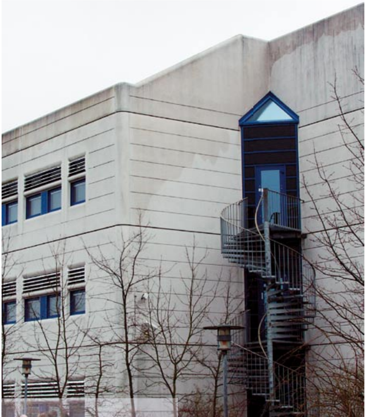
Dirty water running off the roof and onto the facades of an industrial complex, Hørsholm, Denmark.
