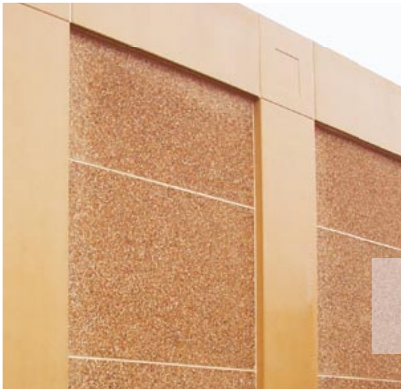
Yellow exposed aggregate and acid-etched surfaces made from one concrete composition, in wet conditions.
