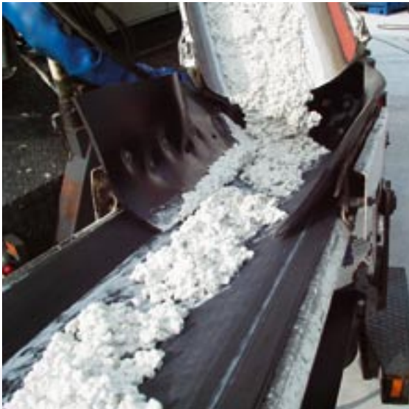
Placing concrete with feeder belt for in-situ cast bridge parapet in Aalborg Denmark.
