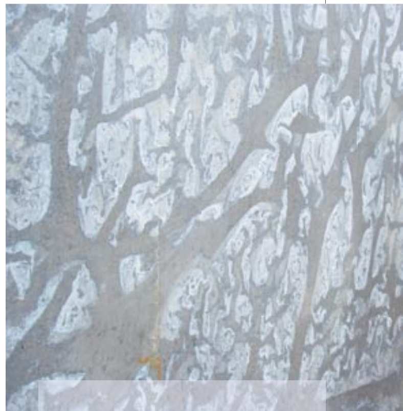
Surface covered with plastic during curing, resulting in areas of varying porosity.
