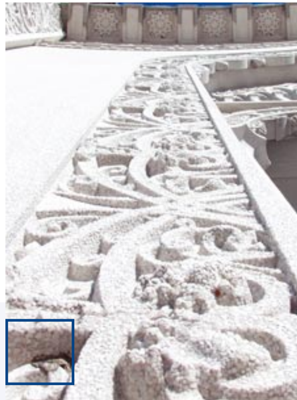
Repair patch made with a different material, neither, matching the colour nor the texture, but only visible from less than 1 metre away. Viewing distance should also be taken into account. The Baha'i Temple, Chicago, Illinois USA.
