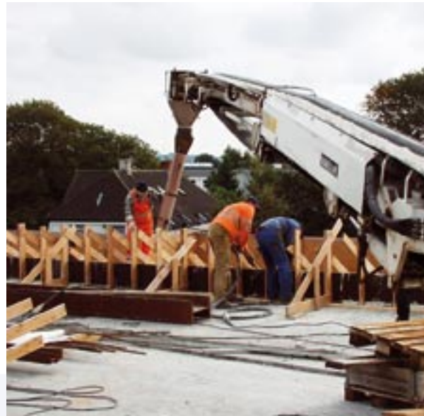
Placing concrete with feeder belt for in-situ cast bridge parapet in Aalborg Denmark.
