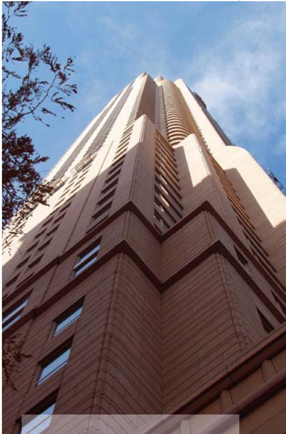
Detail elements at Hyatt Tower, Chicago Illinois, USA: extended projections, small projections, grooves and changes of plane.
