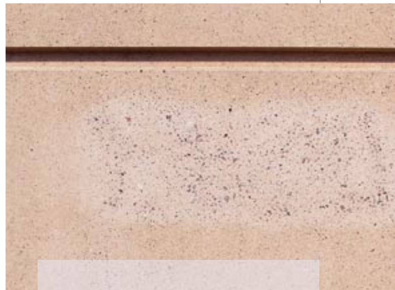
Acid-etched washed surface without coating, after removal of graffiti. Parken, Copenhagen, Denmark.
