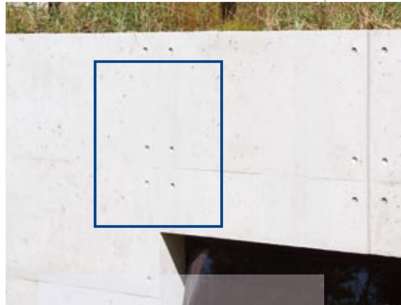
Repair matching both colour and texture of original surface. Distance approx 5 metres. The Bunker Museum, Hanstholm, Denmark.
